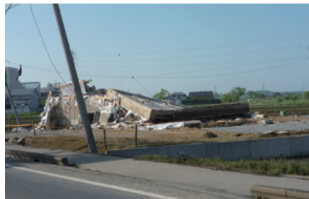
Photo 4: A wooden house overturned with its foundations still attached
