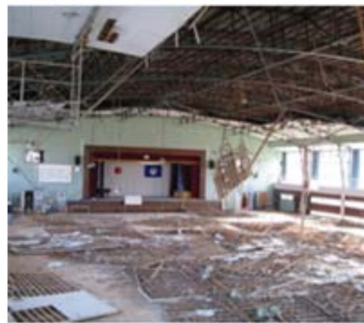
Dropping of extensive ceiling materials and exterior finish materials
