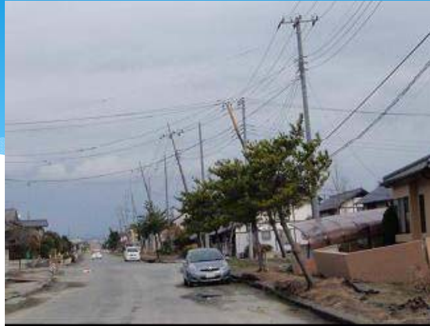
Large-scale liquefaction and settled or tilted structures
