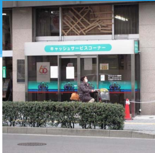
Failure of glass
