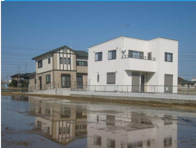
Large-scale liquefaction and settled or tilted structures
