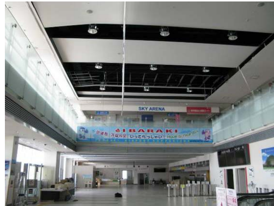
Damage and fall of suspended ceiling
