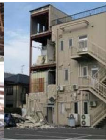
Dropping of extensive ceiling materials and exterior finish materials
