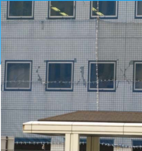
Cracking and spalling of tile
