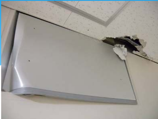
Damage to cover-panels for fire protection
