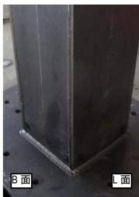
(i) B-L 面柱脚部詳細
